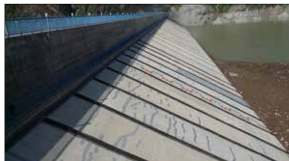
Surface flexible sealing of concrete panels at Jilintai, Xinjiang
