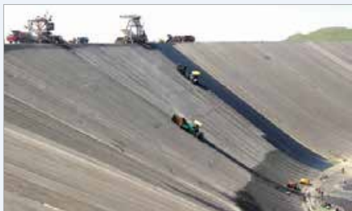
Construction of bituminous concrete face for the upper reservoir of Hohhot Pumped-Storage Power Plant in Inner Mongolia
