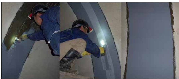
PCCP socket seepage treatment on the Beijing section of the middle route of the south-to-north water diversion project
