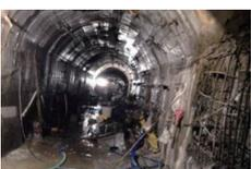
IWHR effectively controls water bursts in a diversion tunnel of hydropower station, overcoming difficulties of cracks, large flow, high pressure, and short distance between bursts and springs
